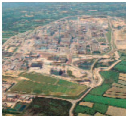
Aerial view of the AREVA fuel reprocessing plant at La Hague.
