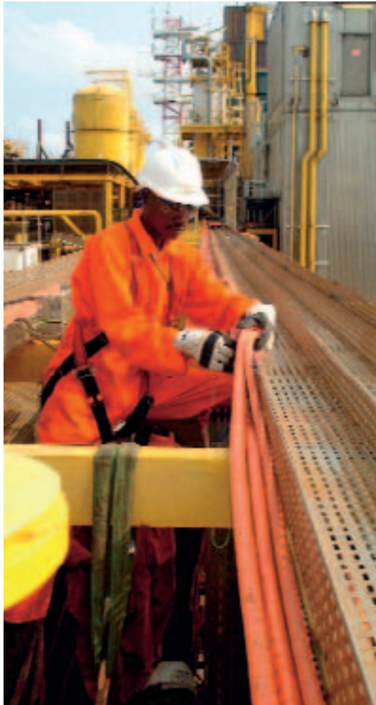
Cable pulling at sea.
