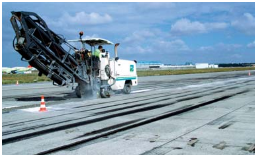
Sawing the ground for the runway shoulder widening operation.
