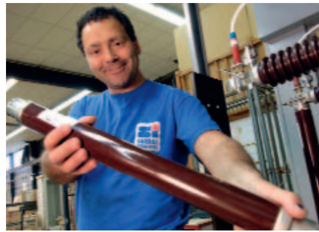
José Pinheiro fits fuses in the 30 kV measuring cell for the Tchibouela site. ▼
