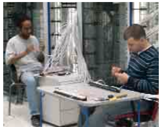
Connecting an RJ 45 plate.
