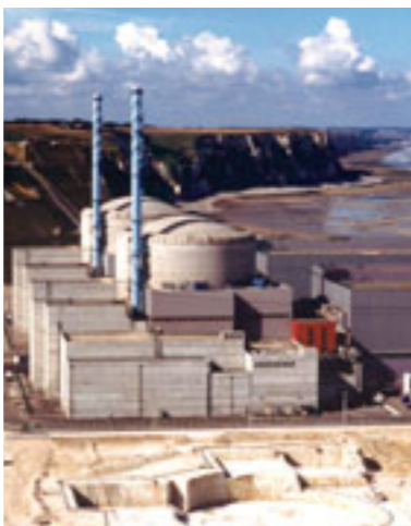
EDF's nuclear power plant at Penly (Normandy).
