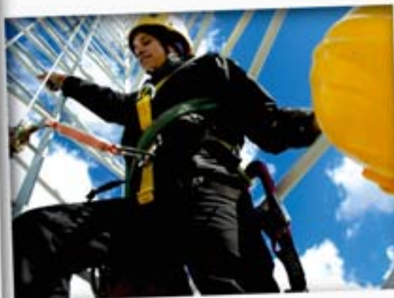
ANOTHER FULLY-EQUIPPED TECHNICIAN, JOHNNY HONDIJK, FOLLOWS DANIEL'S CLIMB TO THE TOP OF THE PYLON SOME 37.5 METRES ABOVE THE GROUND.
