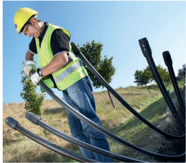
Preparing junctions for the high-density polyethylene tubes.
