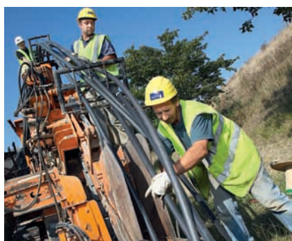
Fitting high-density polyethylene ducts on trench hoes.
