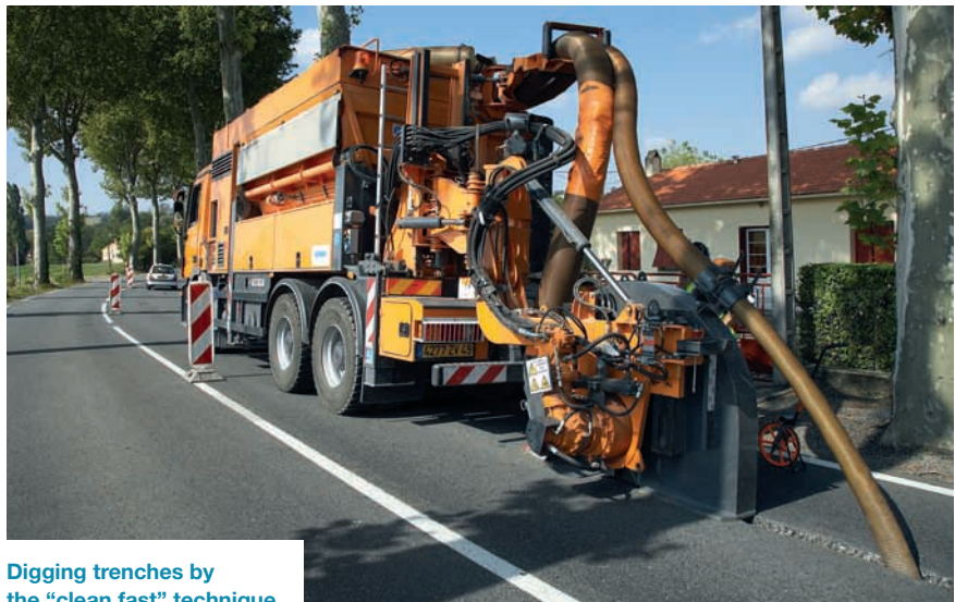
Preparing junctions for the high-density polyethylene tubes.
