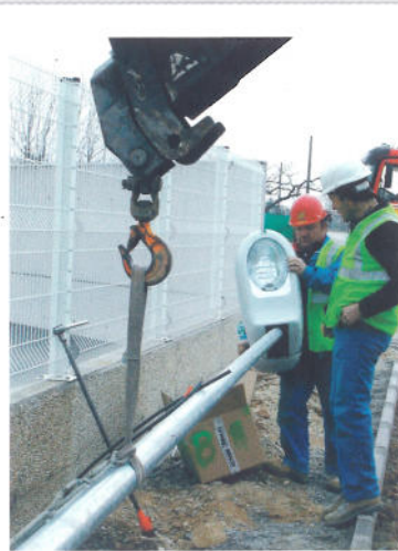
A LAMP-POST READY TO BE LIFTED INTO POSITION BY CHRISTIAN'S LORRY.
