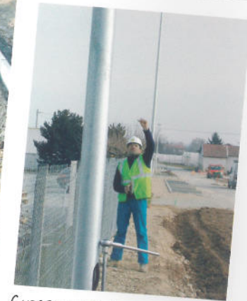
CHRISTIAN USES A PLUMB LINE TO CHECK THAT THE LAMP-POST IS VERTICAL.
