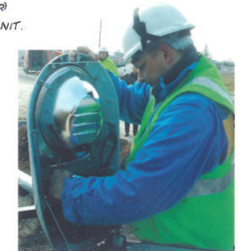
HUGO MOUNTS THE LAMP AT THE TOP OF THE LAMP-POST.
