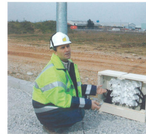
CLAUDE CHECKS A COMPLETED FALSE DISCONNECT CABINET.
