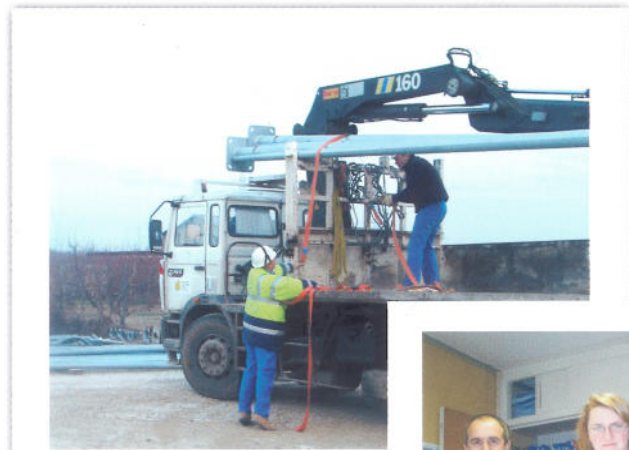
7.30 AM. THE EQUIPMENT IS LOADED AT EEUR'S CENTRE IN MALISSARD.
